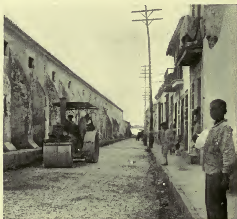
FACTORIA STREET, UNDER REPAIR
